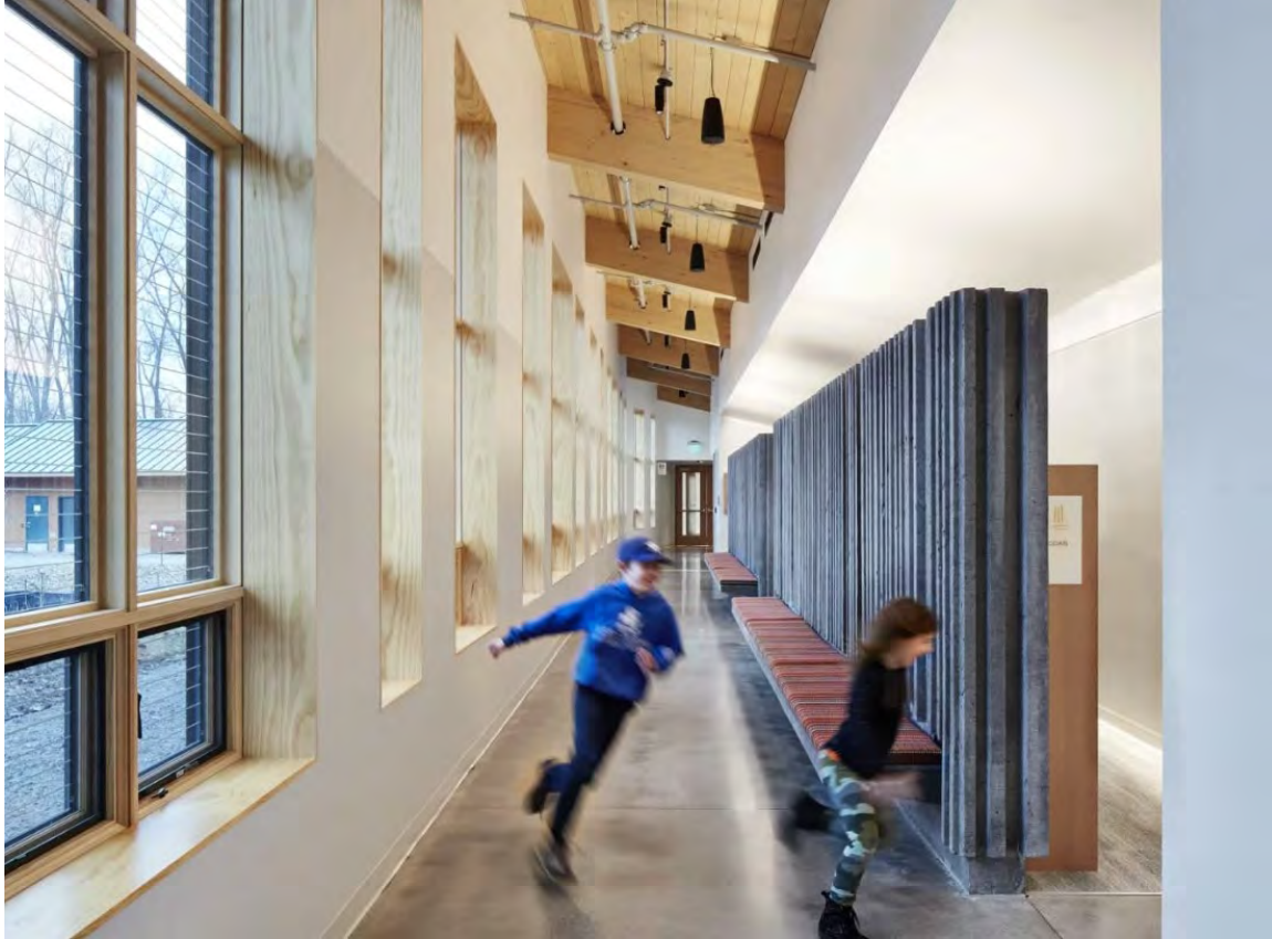
Above: Custom-formed concrete thermal feature walls
