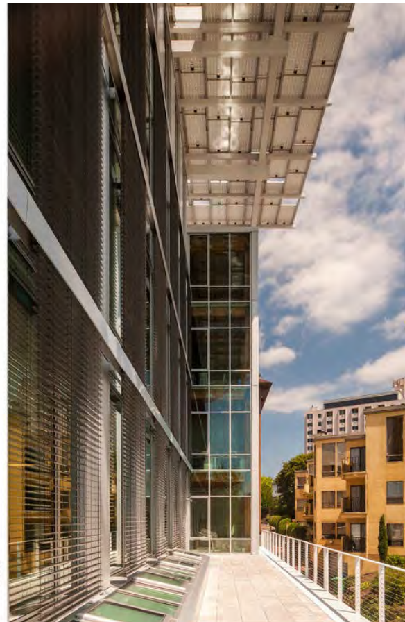
West facade with exterior motorized shades on upper stories. Ground floor is shaded by the trees in the park
