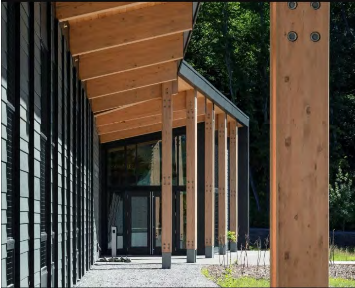
Above: Glue-laminated members exterior covered space
