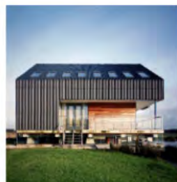
Clerestories and Skylight
